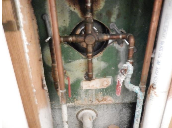
After: New valve and shut off
