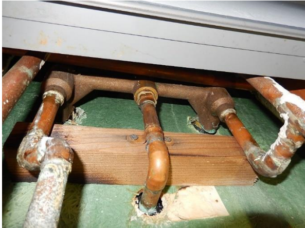
Before: No shut off valve
