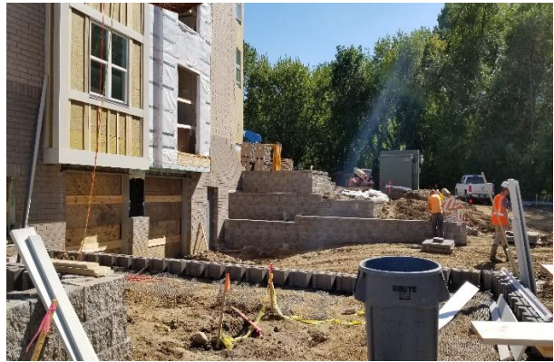
Retaining Walls at Garage Drive
